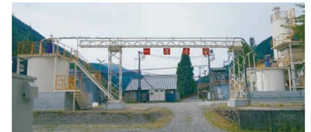
The newly installed milk of lime supply equipment and emergency generators
