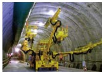
Used for tunneling through mountains in road and railway construction projects in Japan, tunnel drill jumbos dominate the domestic market.
