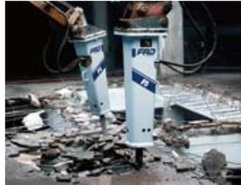
Hydraulic breakers, which are attached to hydraulic shovels, are used for excavating rock and breaking concrete.
