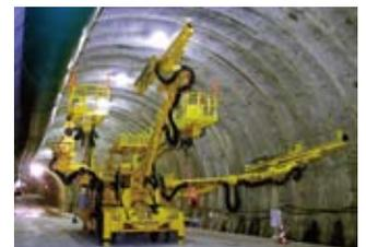
Used for tunneling through mountains in road and railway construction projects in Japan, tunnel drill jumbos dominate the domestic market.
