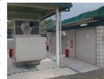
A new fuel storeroom at the Ashio Mine
