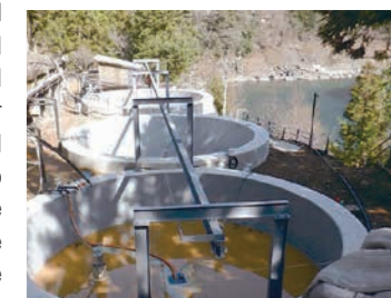
New sludge tanks at the Kune Mine
