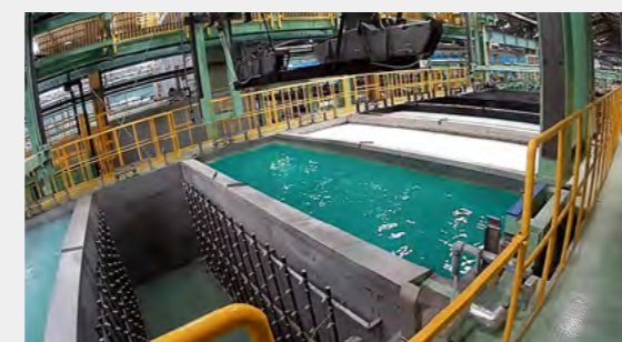
Cationic electrodeposition coating equipment (Sakura Works of Furukawa UNIC Corporation)
