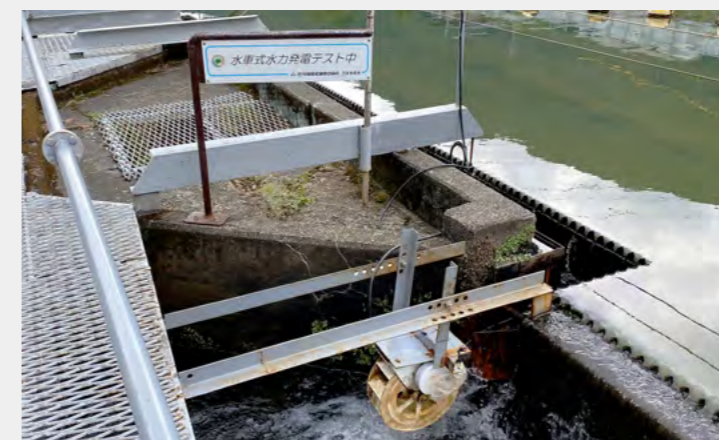
Small-scale hydropower generator (interior of Nakasai Water Treatment Plant at our Ashio Office)
