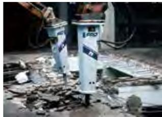
Hydraulic breakers attached to a hydraulic shovel
