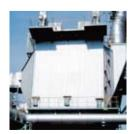
Electrostatic precipitators used for removing particulates from gas emissions and dust from the environment
