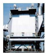
Electrostatic precipitators used for removing particulates from gas emissions and dust from the environment.
