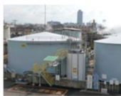
Manufacturing plant of sulfuric acid
