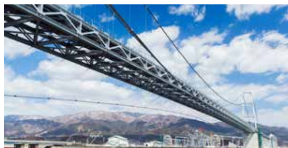
Long-distance belt conveyors adopted for relocation works to higher ground in Rikuzentakata City
